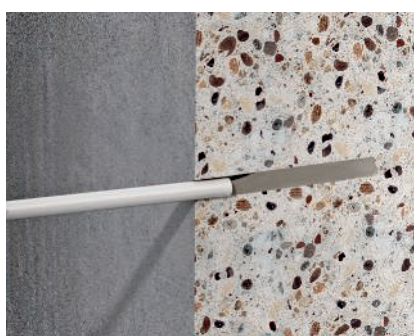
Application of the injection mortar Pressing of the injection mortar into the drill hole.
