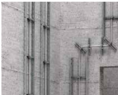
Illustration of vertical shaft Illustration of complete vertical ladder mounting.
